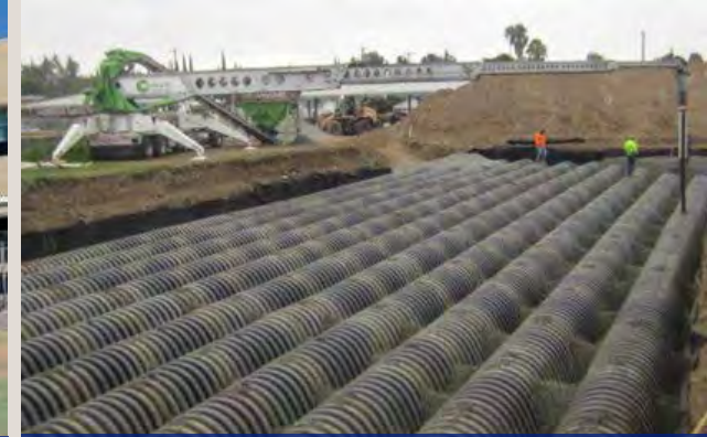
Chatsworth HS – Storm Water Infiltration Basins
