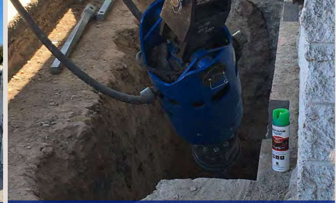
74 th ES – Helical Pile Foundation Underpinning
