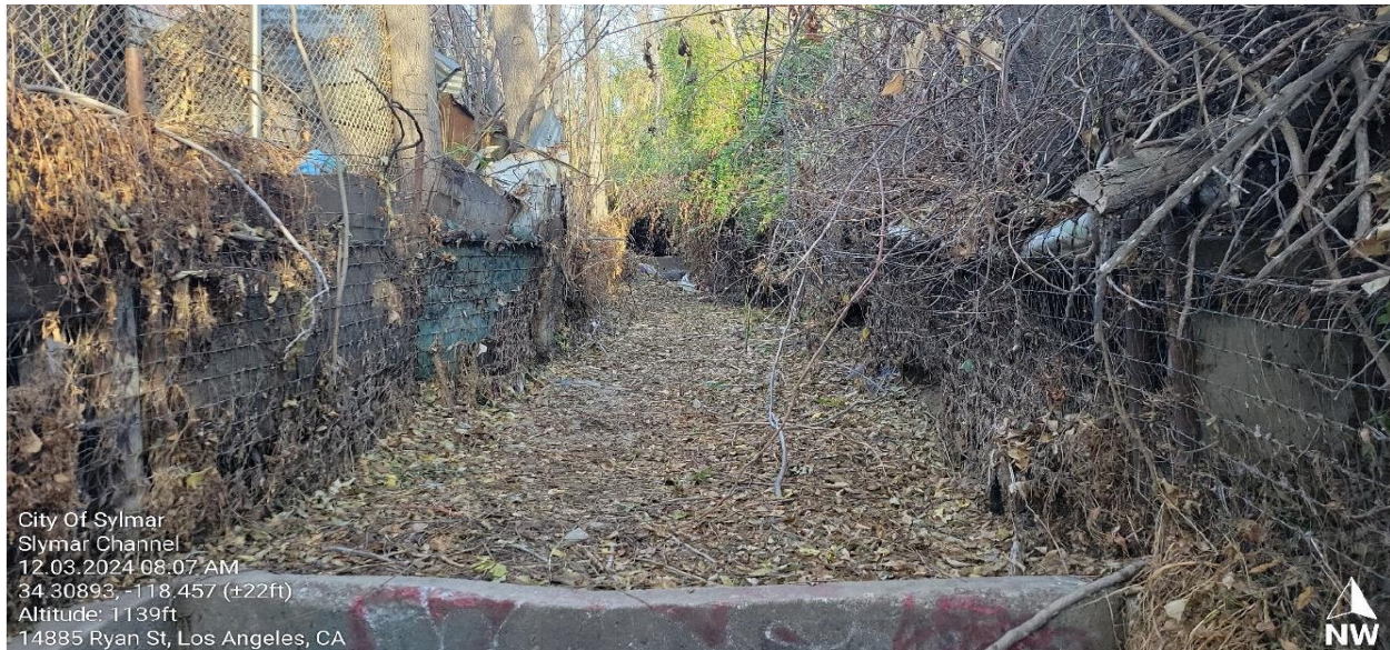
Figure 3. Current channel conditions - central portion looking northwest.
