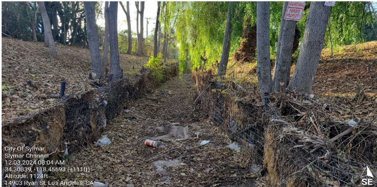
Figure 6. Current channel and bank conditions - southern portion looking south.
