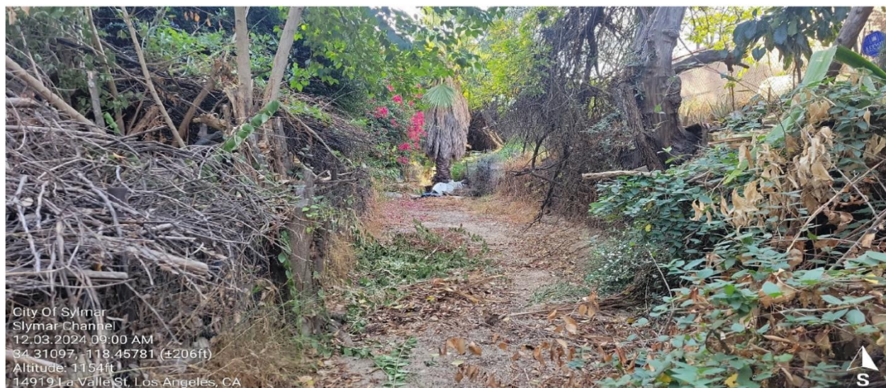
Figure 4. Current channel conditions - central portion looking south.
