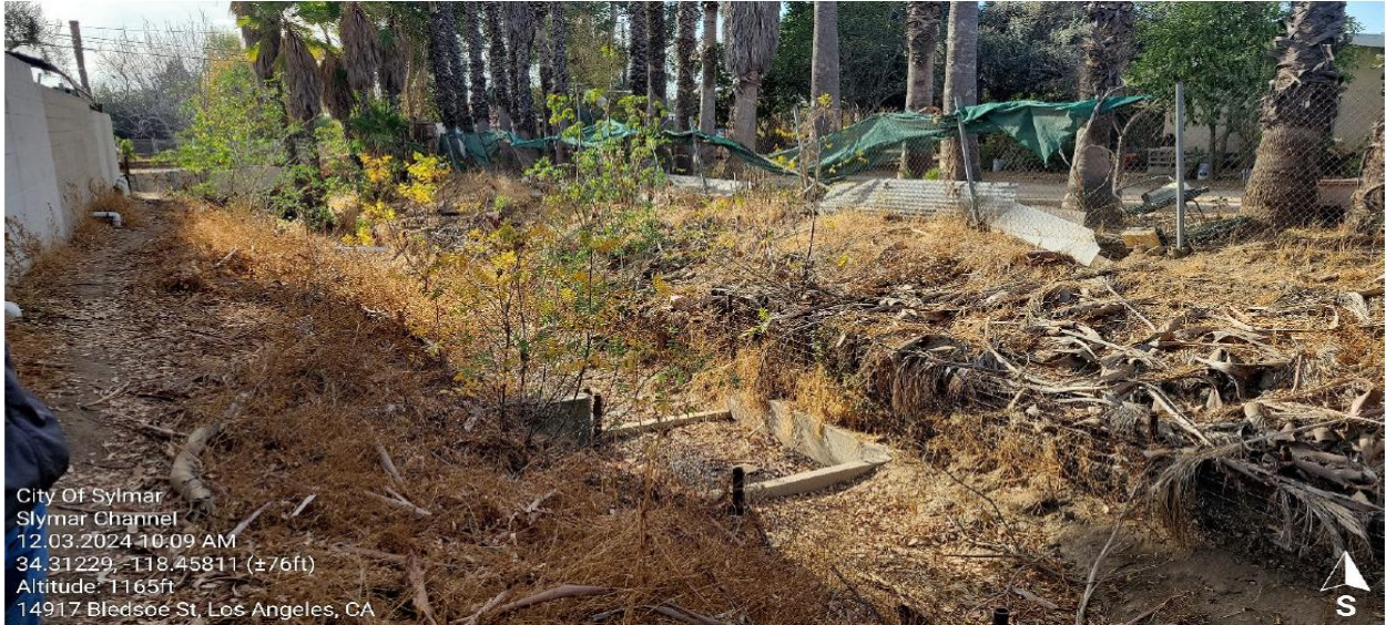
Figure 5. Channel and bank with example of adjacent private residences.
